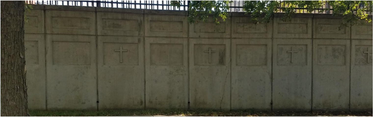
Above is Before Cleaning the wall and After Pictures
